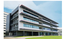
ZEB testing facility “SUSTIE”
