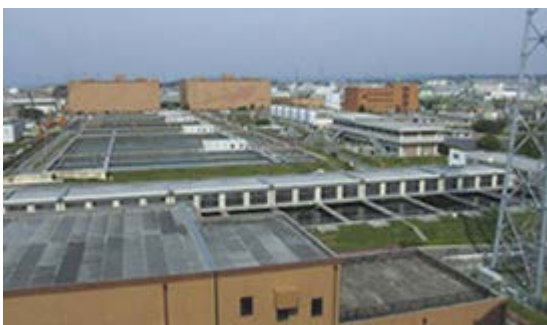
Ozone generator delivered to the Murano Water Purification Plant in Osaka
