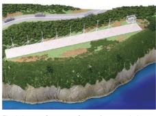
Fig. 1 Image of ocean surface radar transmission and receiving antennas
