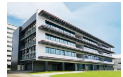
ZEB testing facility “SUSTIE”
